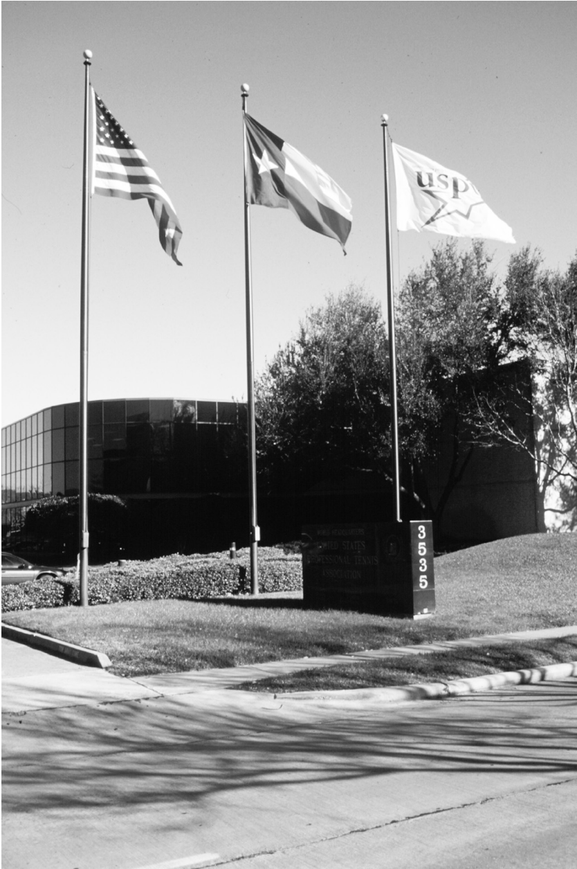
USPTA's World Headquarters building in Houston.
